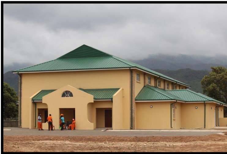
Moshate Community Hall
